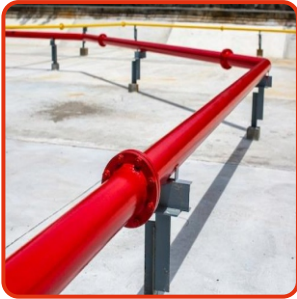
Fire Hydrant Pipeline
